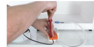
Connection of the LED module to the LED driver and subsequently to mains voltage
