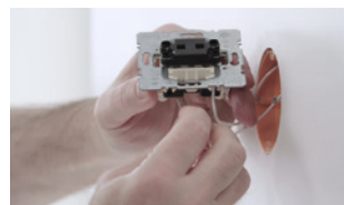
03 Connect the DALI ACU BT to the pushbutton.
