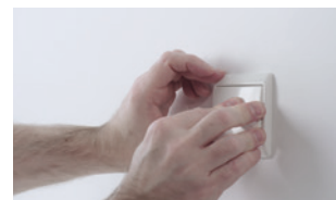
04 Mount the cover of the pushbutton.
